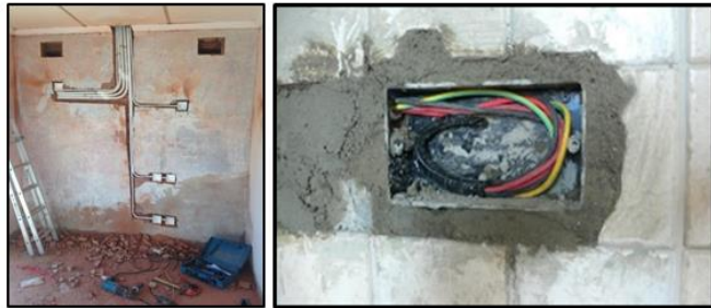
Fig 5.34: Grooves in Brick Wall For Concealed Conduit/Boards Installation
