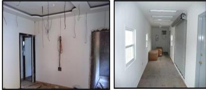
Fig.5.32 Concealed Conduit Wiring Under Construction (Left) & after Finish (Right)
