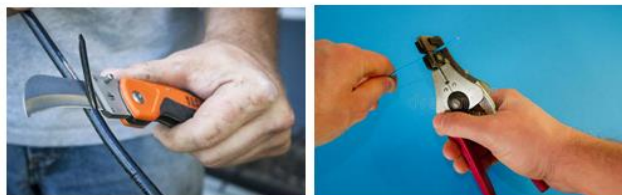
Fig.5.5: Removing the Cable Insulation with Electrician Knife and Wire Stripper
