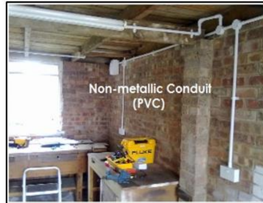
Fig. 5.30: Surface Type PVC Conduit Wiring System
