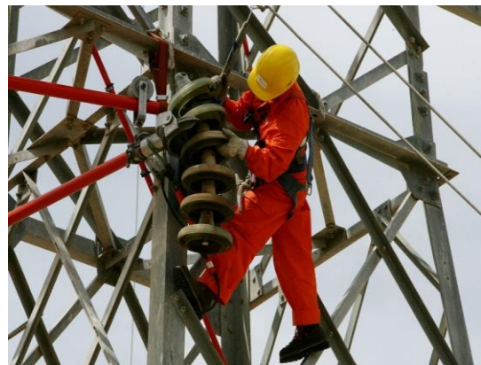
Fig 1.5 Electrical Shock Risk
